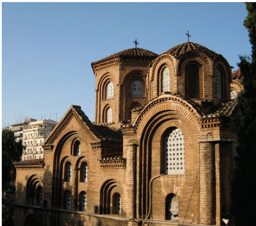
Figure 5.1 Thessaloniki, Panagia Chalkeon, upper part of the south façade from southeast
